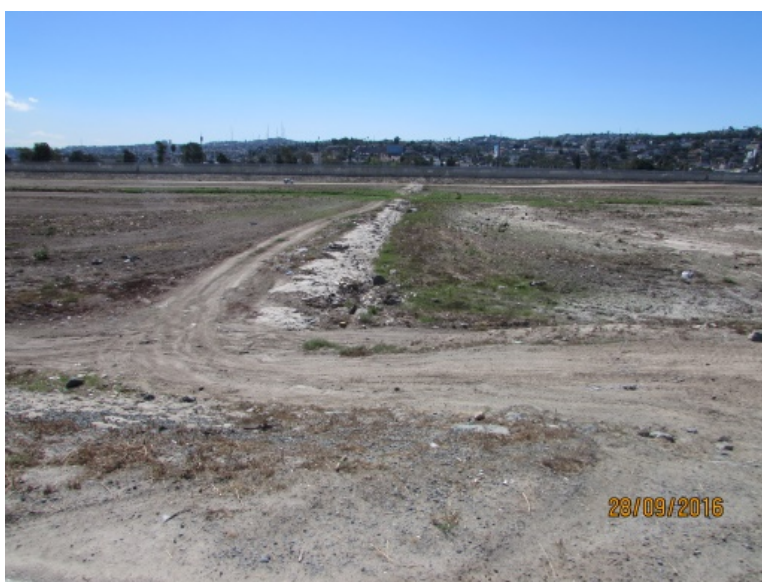
Energy dissipator between the North and South levees.
