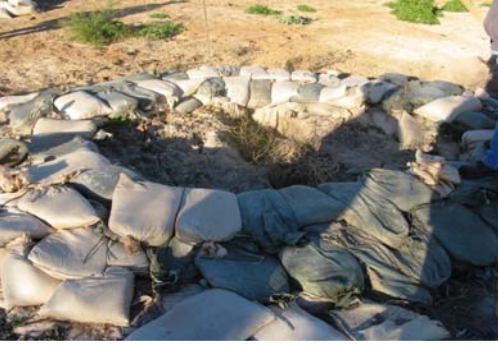
Sand boil near Station 7+000 (picture courtesy George Sills).
