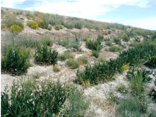
Landside levee slope near geotechnical boring No. 21.
