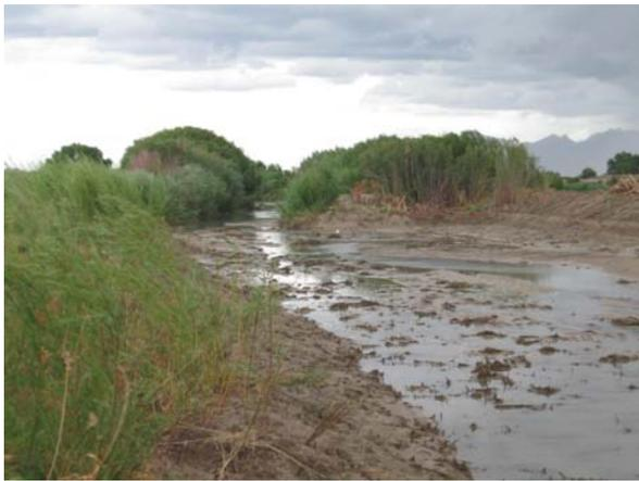
Photo 17: River mile 36. MxIBWC completed dredging operations. Note dense vegetation (primarily salt cedar) along Rio Grande downstream of dredging operations, and widening of main channel.
