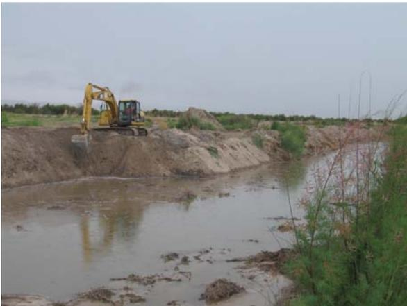
Photo 21: River mile 48-50. MxIBWD dredging operations; note bank cut back of at least 10 feet, and bank vegetation removal.
