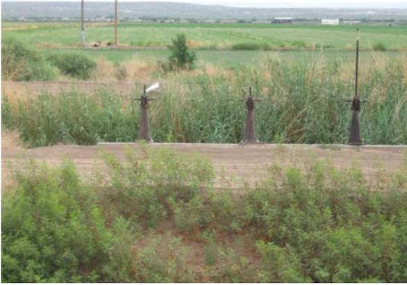
Photo 22: River mile 53.5. Screw gates on landside of levee at Alamo Grade. Snowy egret on left.
