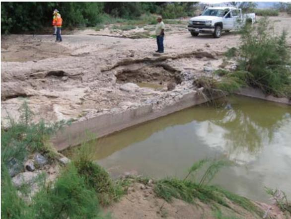
Photo 39: River mile 77.5. Broken Box Culvert Drain.
