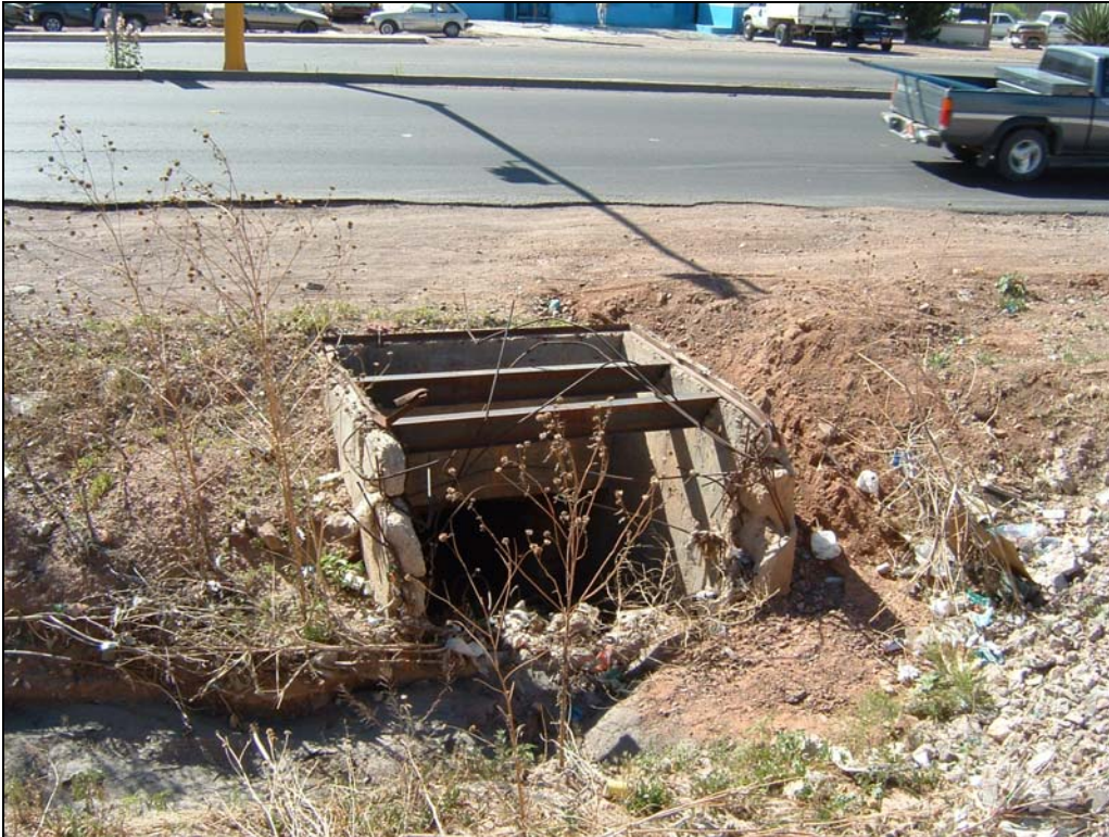
Figure 5. Tributary Inlet for Subarea L1 at International Highway.
