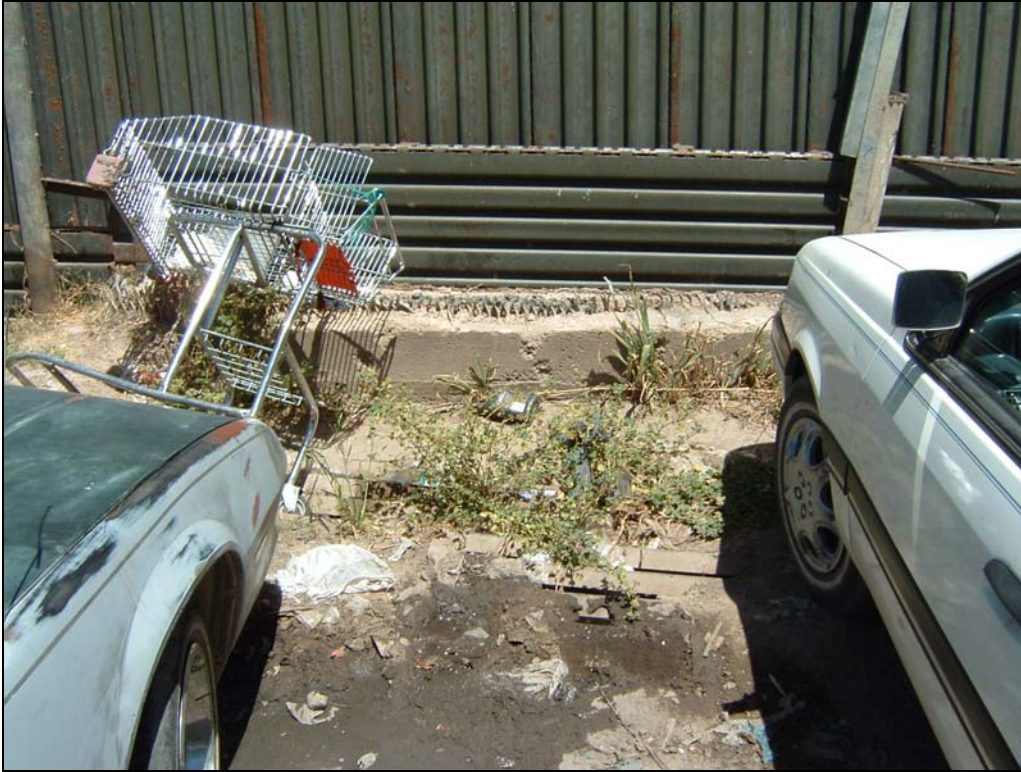
Figure 15. Grated Inlet Structure Along Calle Internacional
