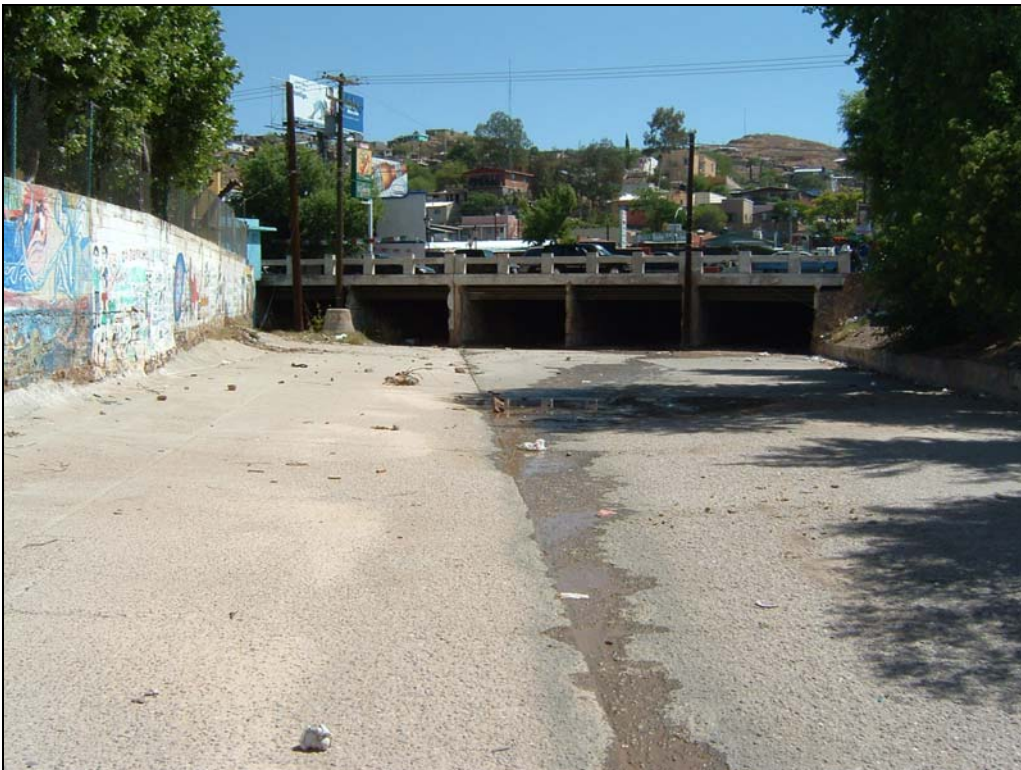
Figure 8. Tributary Inlet for Arroyo Chimeneas
