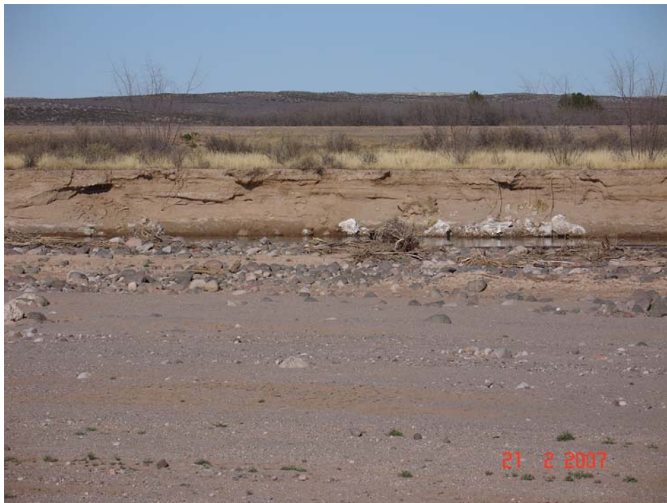
Figure A.6. View east across the Rio Grande at the confluence with Bignell Arroyo showing lateral erosion of the left bank and the RGCP levee in the background.
