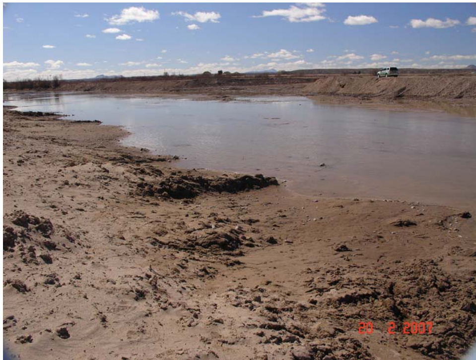
Figure A.37. View downstream of the Rio Grande from the Arrey Bridge showing the channel depth that has resulted from 4 to 6 feet of degradation.
