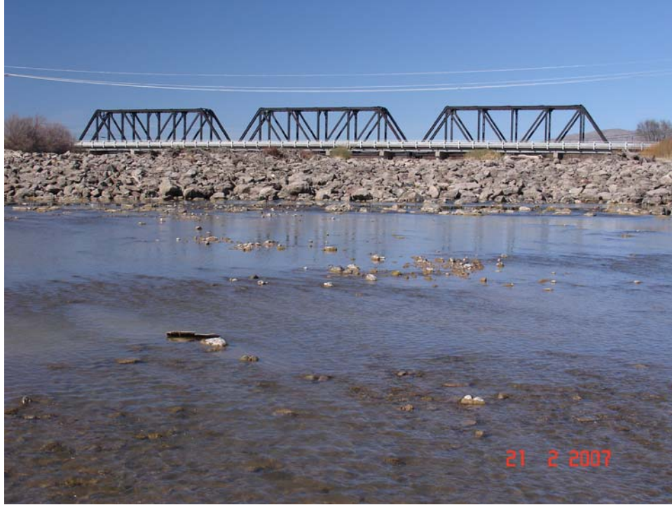
Figure A.45. View upstream of the rock riprap at the Rincon Siphon. In the background are the Highway 140 and BNSF Railroad Bridges.
