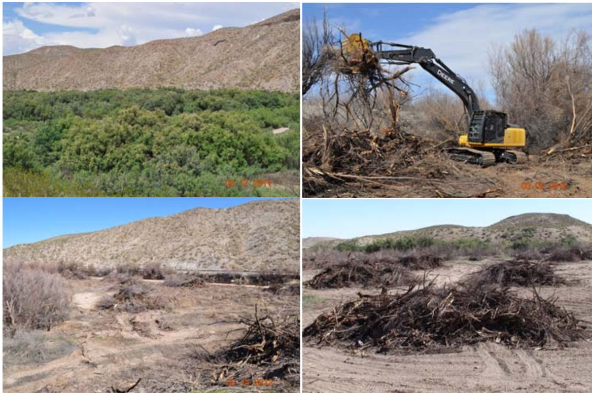
Figure 2-9. Mechanical Excavation Treatment method at the Broad Canyon Arroyo restoration site. A) Top left - example of monotypic stand of saltcedar. B) Top right - equipment excavating saltcedar. C) Bottom left - landscape after excavation. D) Bottom right - debris piles.
