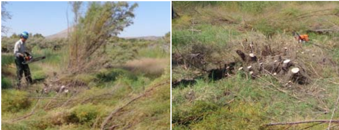
Figure 2-6. A) Left - Manual treatment method involving cutting with chainsaw, and (B) Right - immediate herbicide application on cut stumps.
