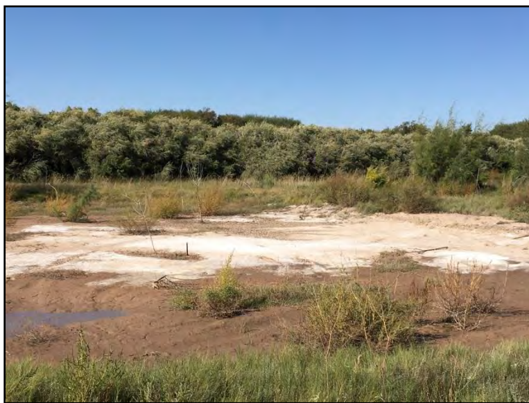
Swale at Country Club East with some salt accumulation, 16 October 2019.
