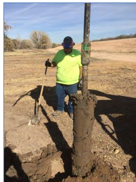
Augering holes for cottonwood pole planting at Sunland Park, 21 March 2018
