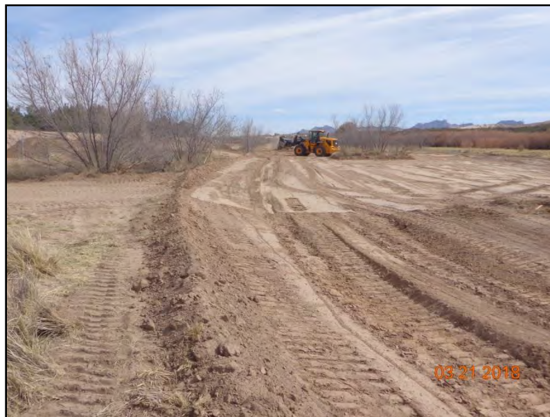
Creating the drainage swales created at Country Club East, 21 March 2018.
