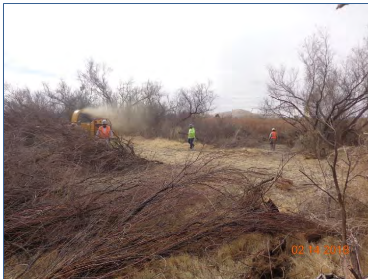
Saltcedar extraction and chipping at Sunland Park, 14 February 2018
