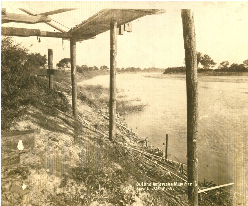
Figure 3.9. View of the study area riverbank in 1927 from beneath the frame support for the Gateway International Bridge pier. View is looking downstream and shows a bank slope of approximately 3H:1V.
