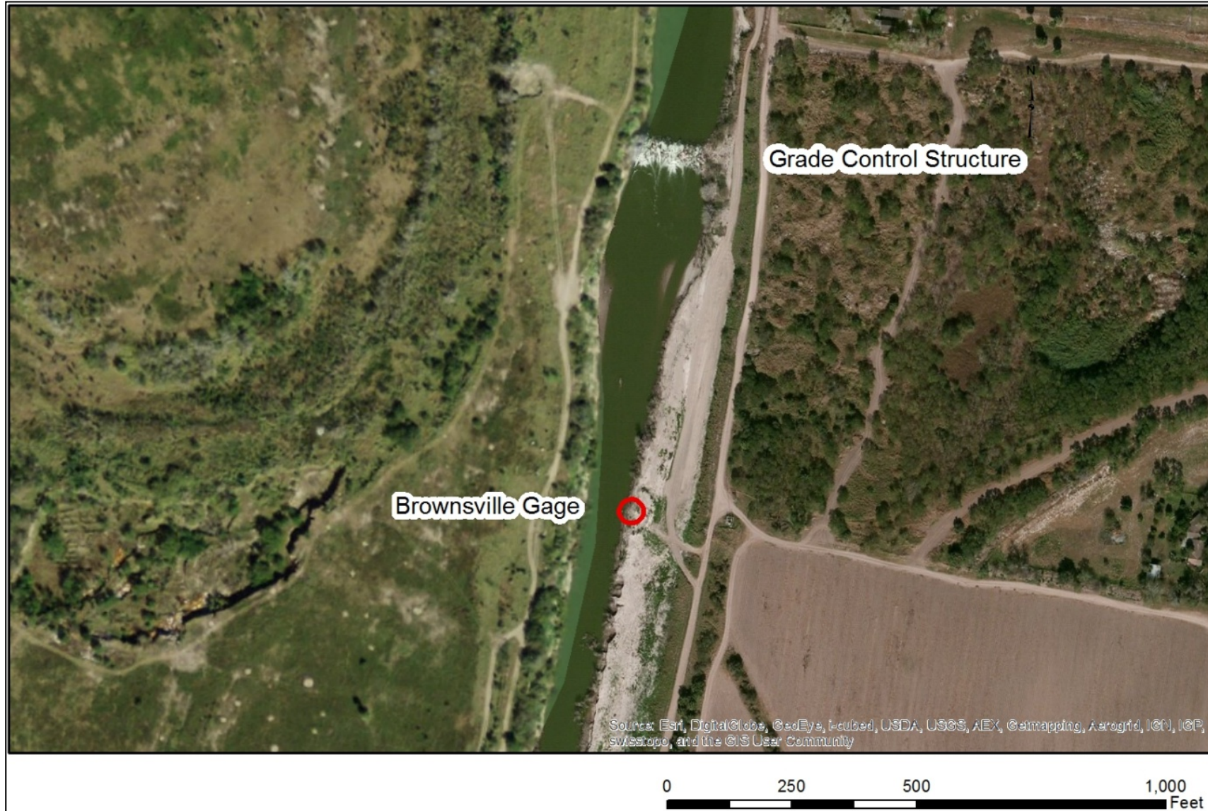
Figure 5.12. Close-up of grade control structure showing rock construction upstream of the gage (2014 Google Earth Image).
