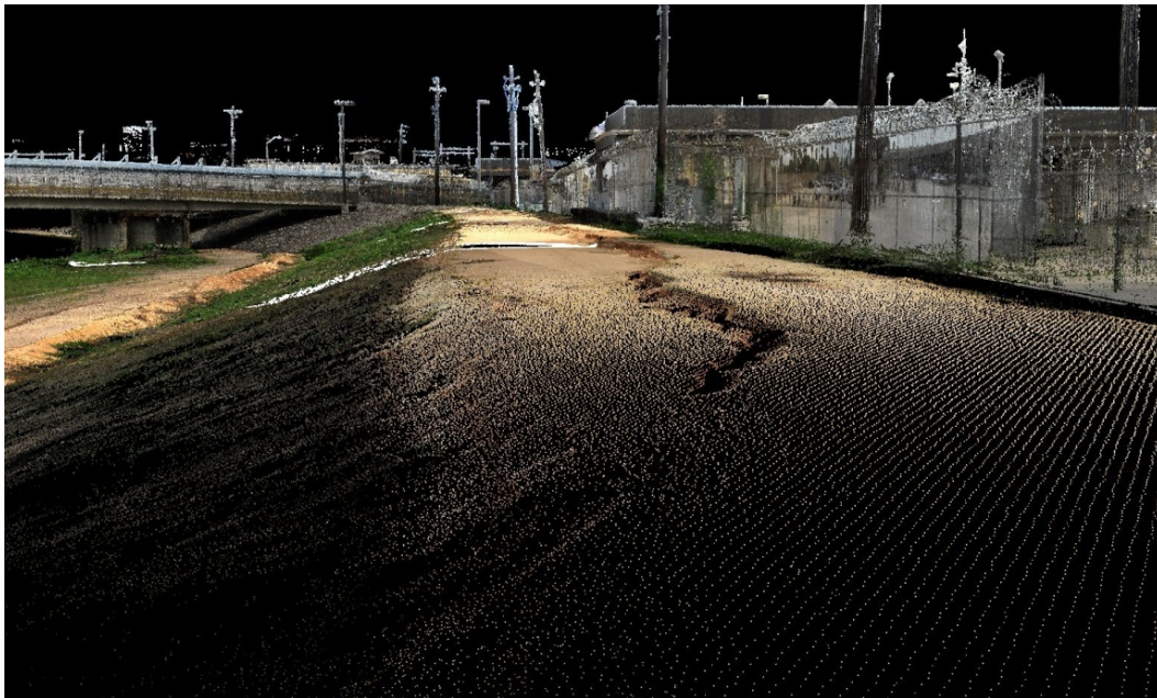
Figure 4.21. LiDAR image looking upstream and showing 0.5 to 0.7 ft of down slope displacement of the crest road.
