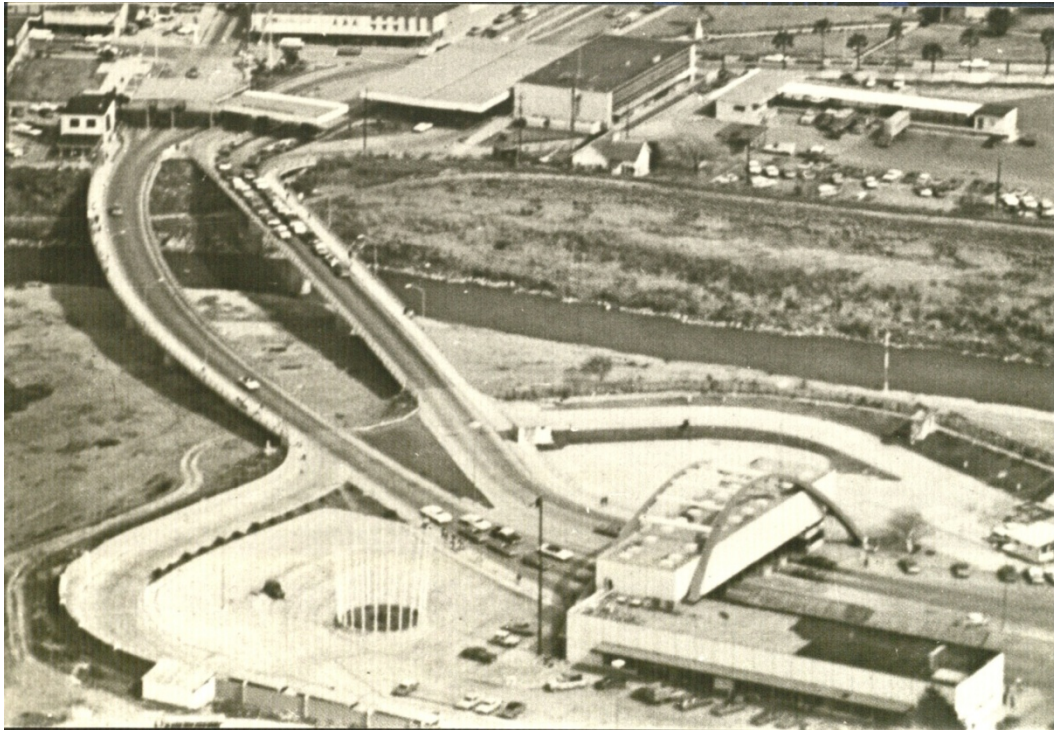
Figure 3.13. View of second Gateway International Bridge from Mexico approximately late 1960s or early 1970s (courtesy of Brownsville Historical Society).
