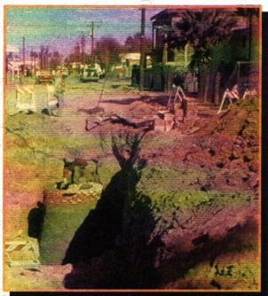
The majority of the small-diameter sewer collector improvements requires the contractor to reconstruct or build new access manholes. These are constructed in-place using clay bricks and mortar. Their height (or how deep they extend into the ground) depends on the depth of the sewer collector.
