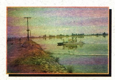
View of a recently constructed earthen basin in the Ignacio-Zaragoza treatment facility receiving dredged sludge from one of its stabilization lagoons. The cement wall shown in the photo is part of the main feeder canal to the facility (which runs along the north end of the property).
