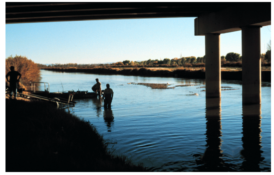
Station 2- Zaragoza Bridge
