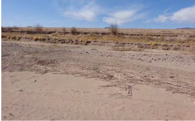
Figure 4-5. Eroded banks encroaching on the levee opposite Rincon Arroyo, looking slightly downstream, March 2013.
