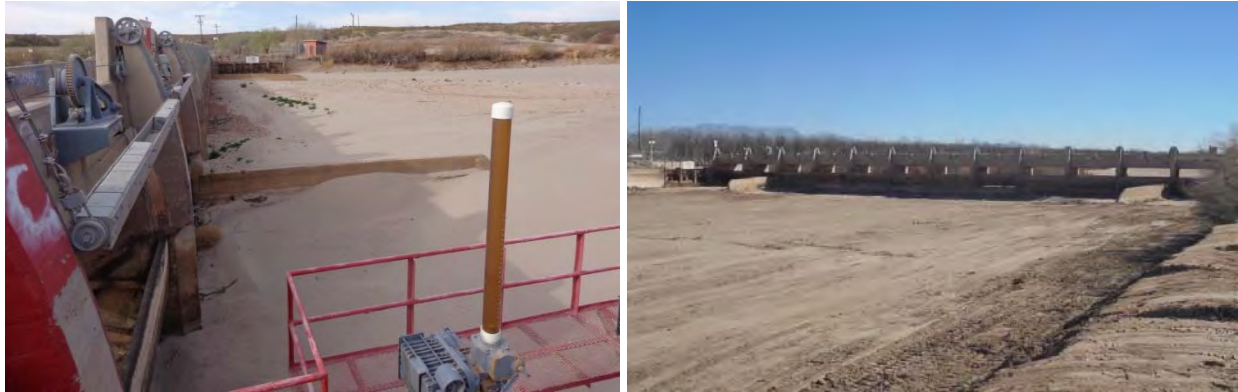
Figure 4-7 Left – Sediment accumulation at Mesilla Dam, March 2013. Right – After excavation, January 2016.
