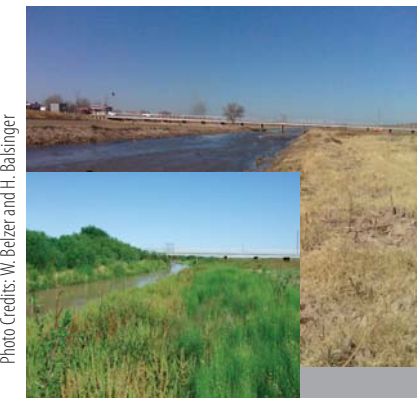
IBWC Minute 313 allows for maintenance of the floodplain and channel to address flood concerns. These photos show Station 15704 in May 2007 (bottom) and in December 2008 (top).
