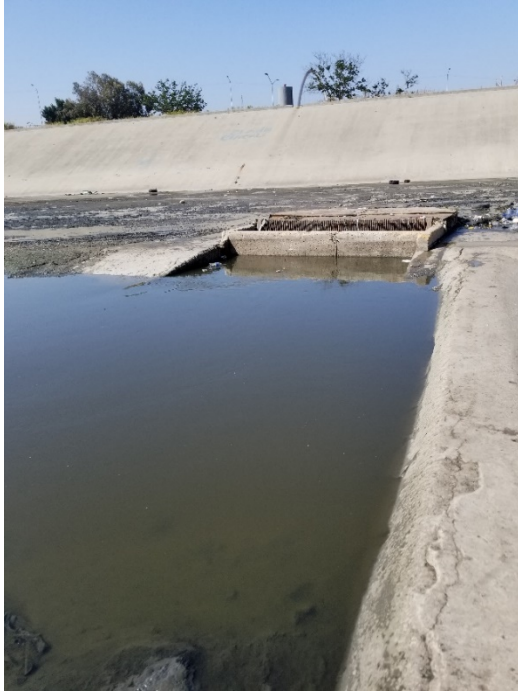
Figure 17. Tijuana River at the PB-CILA diversion structure.
