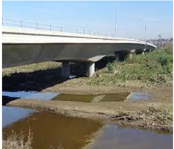
Figure 19. Tijuana River at Dairy Mart Bridge.
