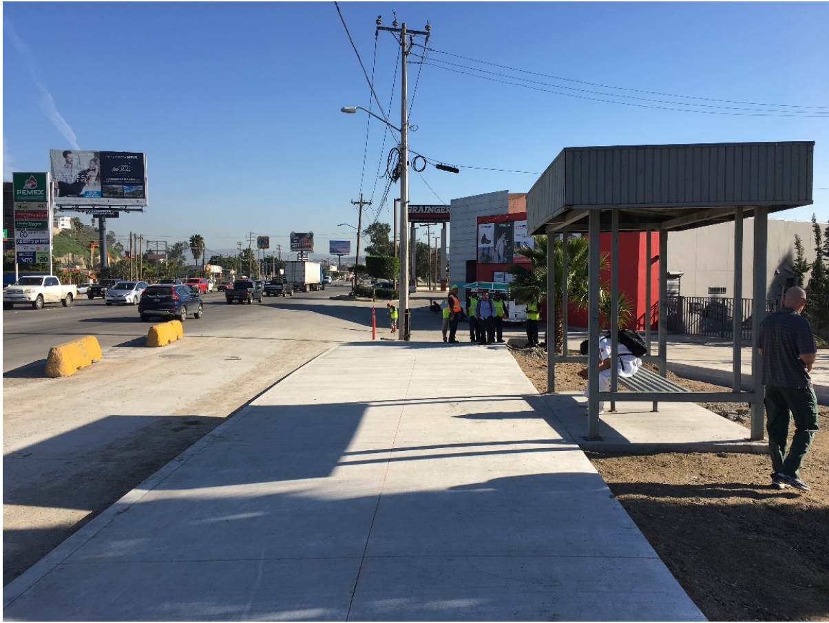
Figure 11 Final repairs to road and bus stop and location of Insurgentes/Oriente collector repair- - Blvd Lazaro Cardenas, Colonia Los Pirules, Tijuana, B.C. - March 9, 2017
