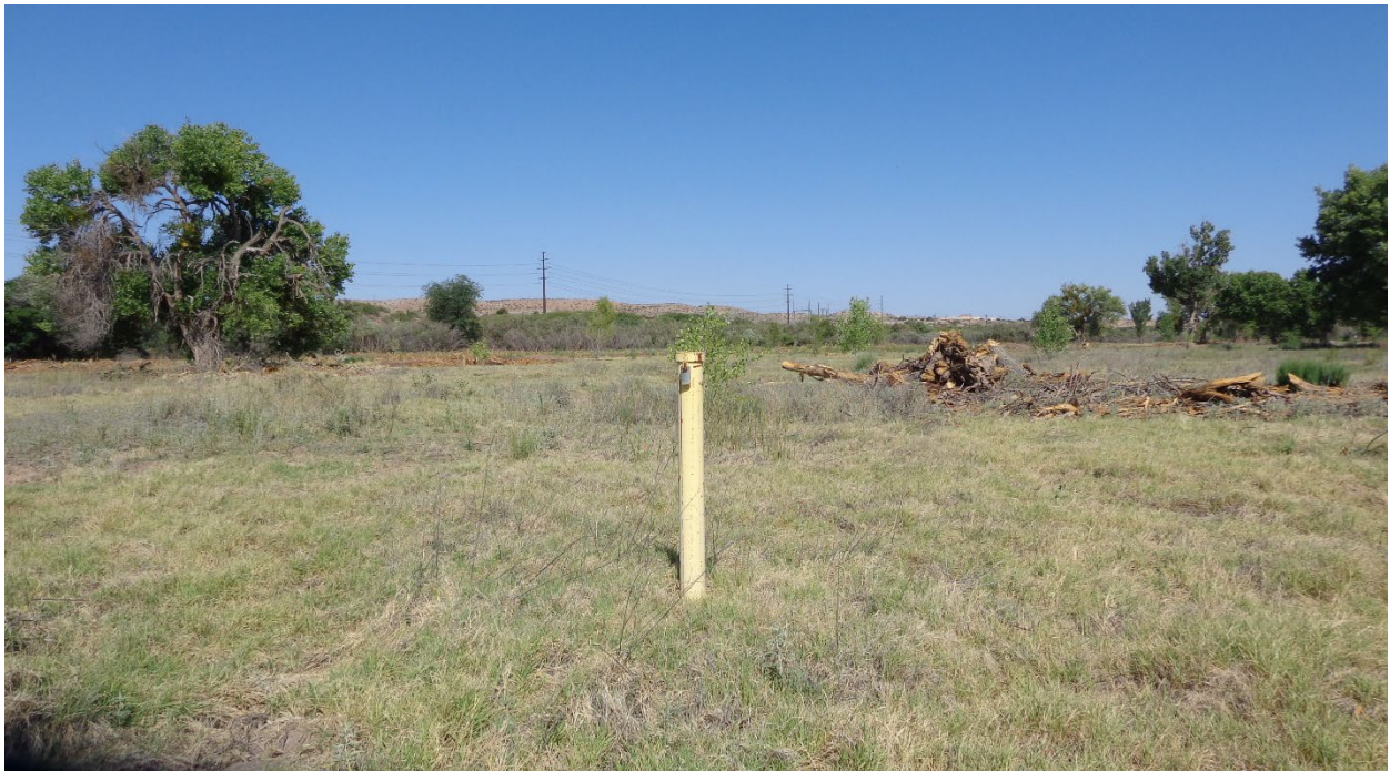
View from well SP-MW-2, tree on the left and wood and bark debris on the right. Some of these trees seem to be dying and a cause of this could mistletoe or some sort of fungal infection.
