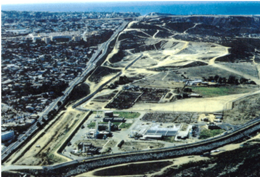
Figure 1. South Bay International Wastewater Treatment Plant
