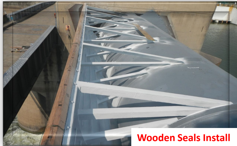
Stoplog Installation
