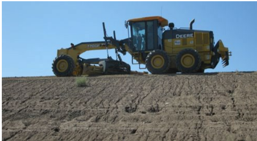
Equipment on the levee
