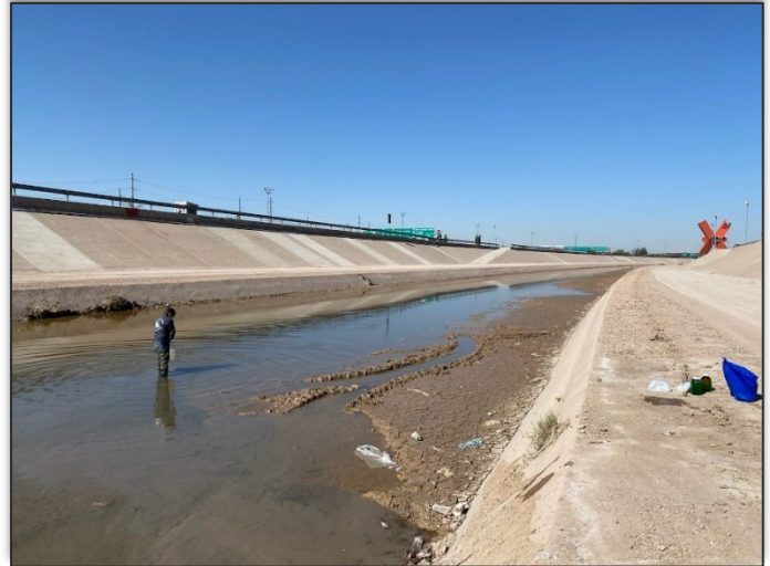
Station 14665 located in the channelized portion of the Rio Grande.
