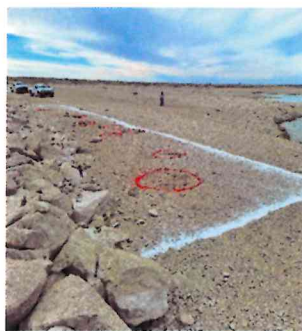
January 30, 2024 The sinkholes identified with consecutive numbers from #40 to #48 were detected in an area at the toe of the upstream slope between km 5+770 and 6+230.
