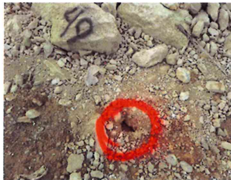
February 07, 2024 The sinkholes identified as #49 and #50 are observed at the toe of the upstream slope of the embankment.
