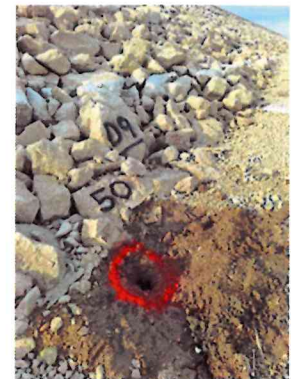
February 07, 2024 The sinkholes identified as #49 and #50 are observed at the toe of the upstream slope of the embankment.
