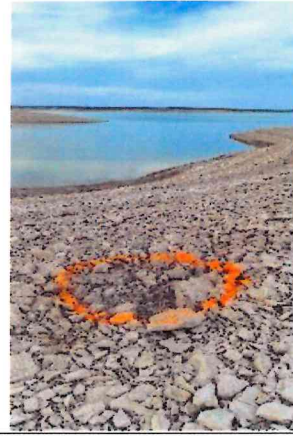
February 26, 2024 Sinkhole #54 located at Station km 5+450 was observed 320 m away from the toe of the upstream slope.
