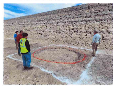
January 30, 2024 The sinkholes identified with consecutive numbers from #40 to #48 were detected in an area at the toe of the upstream slope between km 5+770 and 6+230.
