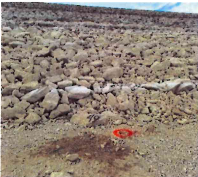
February 07, 2024 The sinkholes identified as #49 and #50 are observed at the toe of the upstream slope of the embankment.
