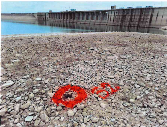
February 16, 2024 Sinkhole #52, located at Station km 5+373, 211 m away from the embankment.
