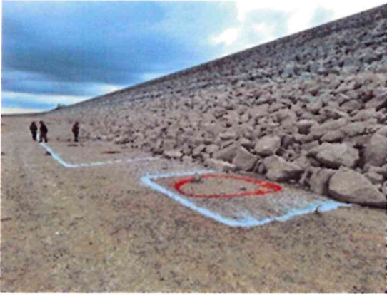
February 08, 2024 A new sinkhole was detected and labeled #51 based on the next consecutive number.
