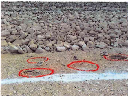
January 30, 2024 The sinkholes identified with consecutive numbers from #40 to #48 were detected in an area at the toe of the upstream slope between km 5+770 and 6+230.
